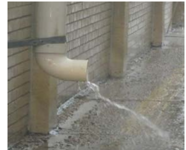
This downspout connects to the roof gutter.
